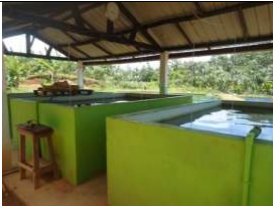
Infrastructure in the hatchery
